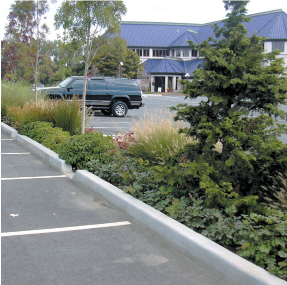
Figure 10. Bioswales play an important role in urban areas, filtering groundwater runoff.
