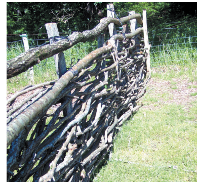
Figures 17. Woven fences are structurally sound and use natural materials, reducing our footprint.
